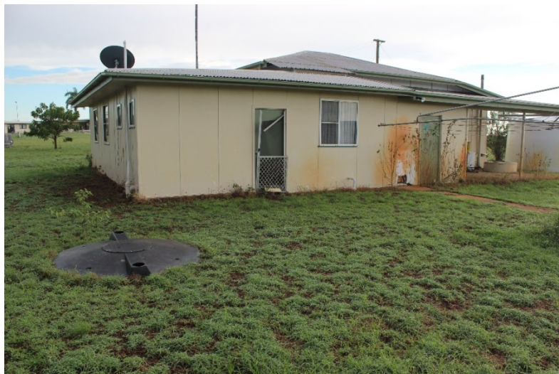
Plate 18-8: ID No. 3: Workers residence rear view and northly aspect
