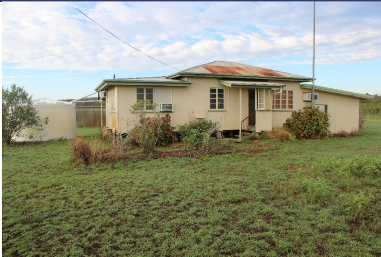
Plate 18-7: ID No. 3: Workers residence front view and southerly aspect
