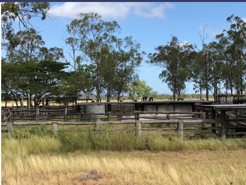
Plate 18-9: ID No. 3: Timber post and slab stockyards
