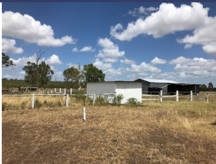
Plate 18-5: ID No. 2: House yards at the rear of the main farm residence north westerly aspect
