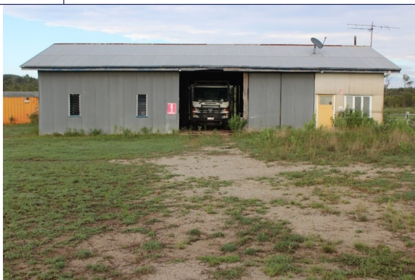
Plate 18-4: ID No. 2: Machinery shed to the west of the main farm residence, easterly aspect
